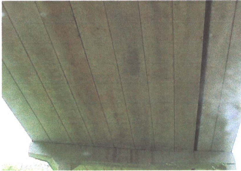
BOTTOM OF DECK
