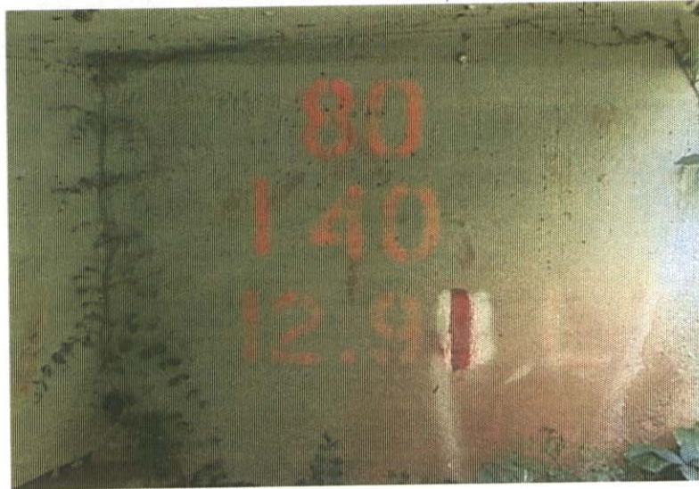
BRIDGE NO. AT ABUTMENT # 1
